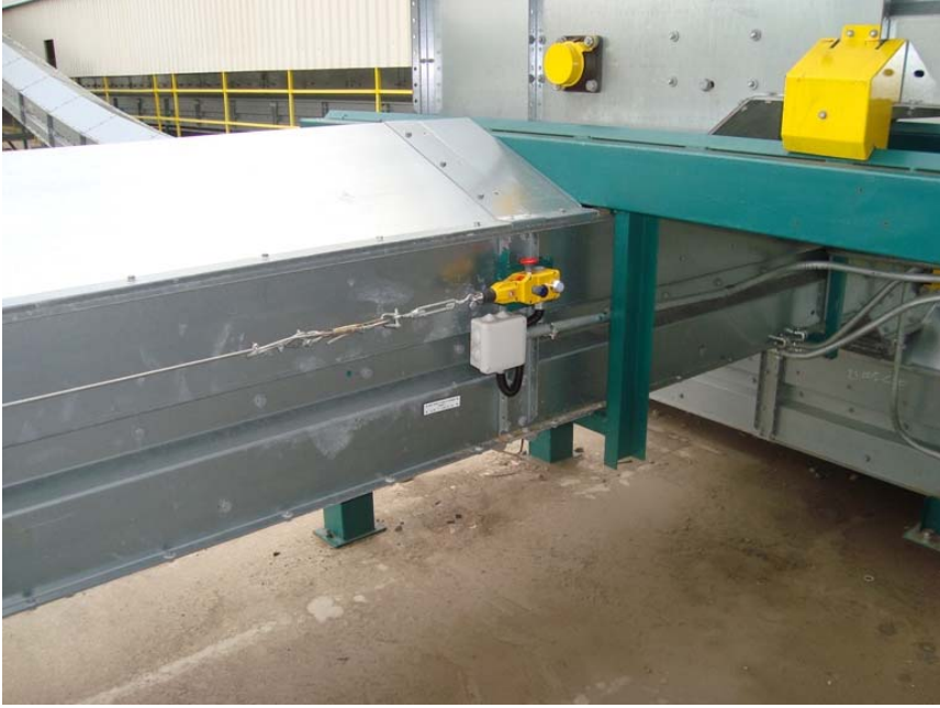
Emergency Pull Cord in MONSANTO Electrical Construction Phase II
