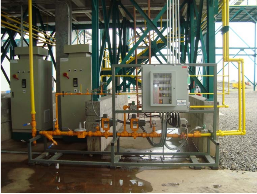
150 HP Blower Motor MCC and Dryer Control Panel in MONSANTO Electrical Construction Phase II
