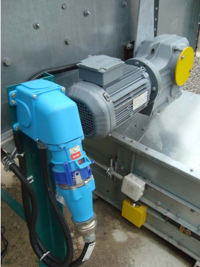
MARECHAL Receptacle Installation in MONSANTO Electrical Construction Phase II
