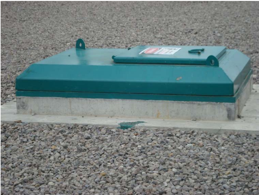
Pull Box for pulling cable power
