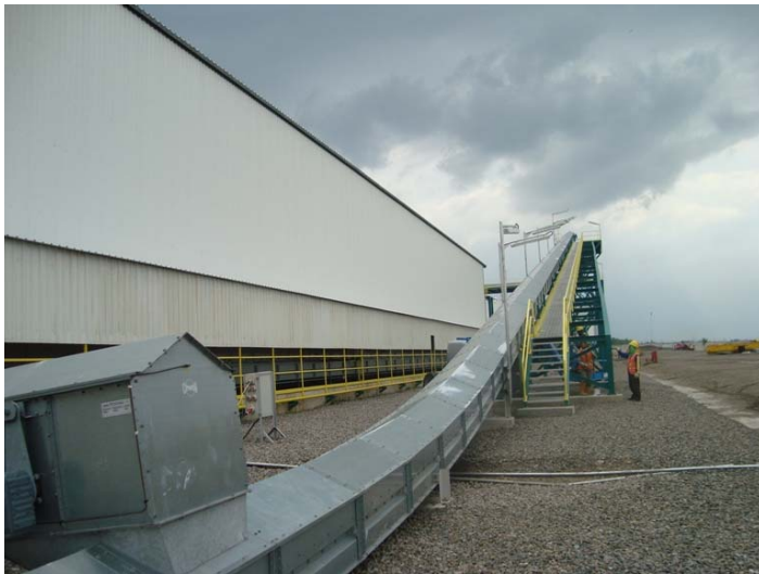
Lighting for Cross Yard Conveyor
