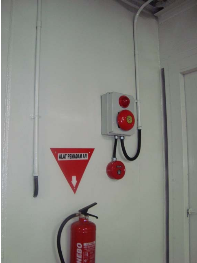
Fire Alarm System Installation
