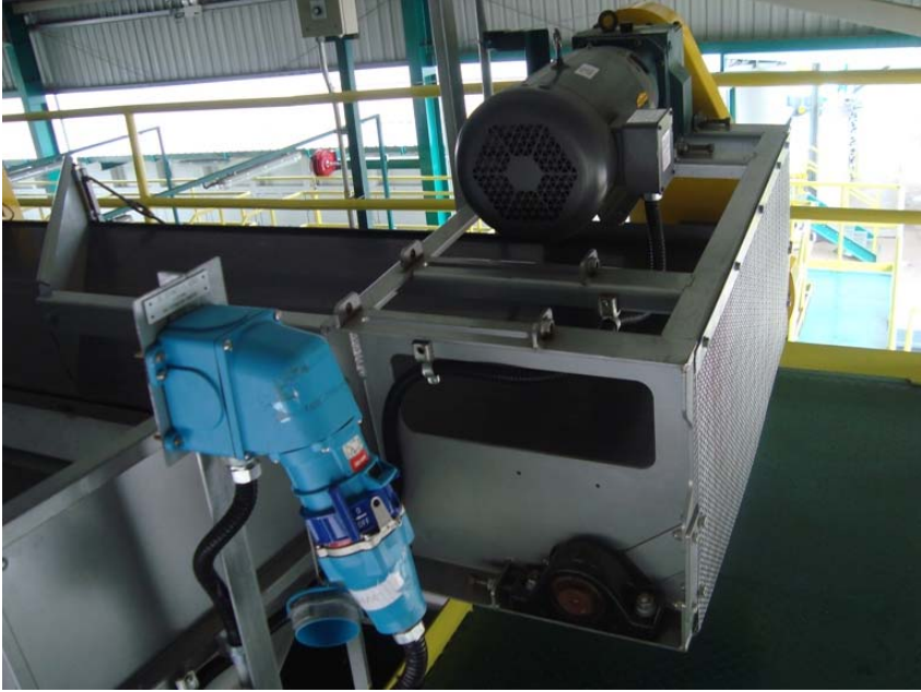
MARECHAL Receptacle Installation in MONSANTO Electrical Construction Phase II
