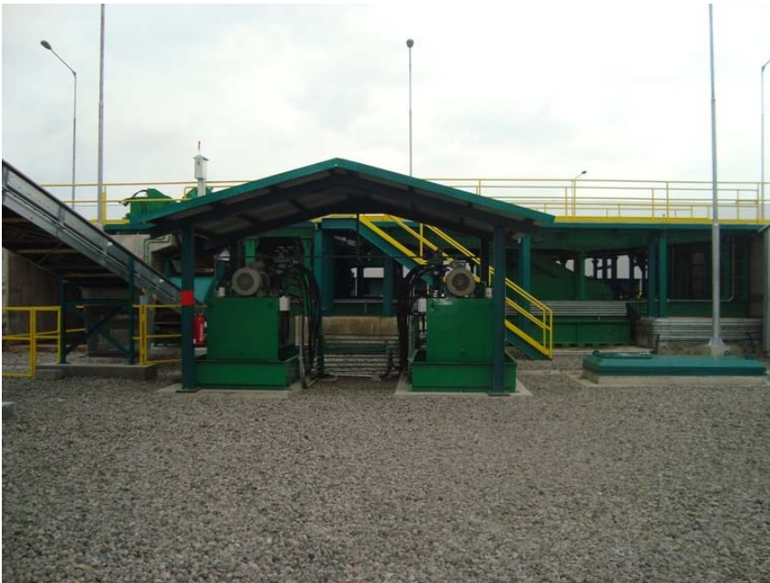
Truck Tripler Hydraulic Motor Pump in MONSANTO Electrical Construction Phase II
