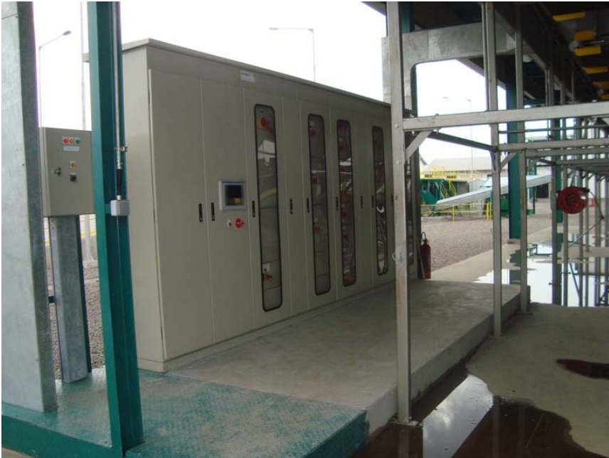
Green Corn Sorting MCC in MONSANTO Electrical Construction Phase II
