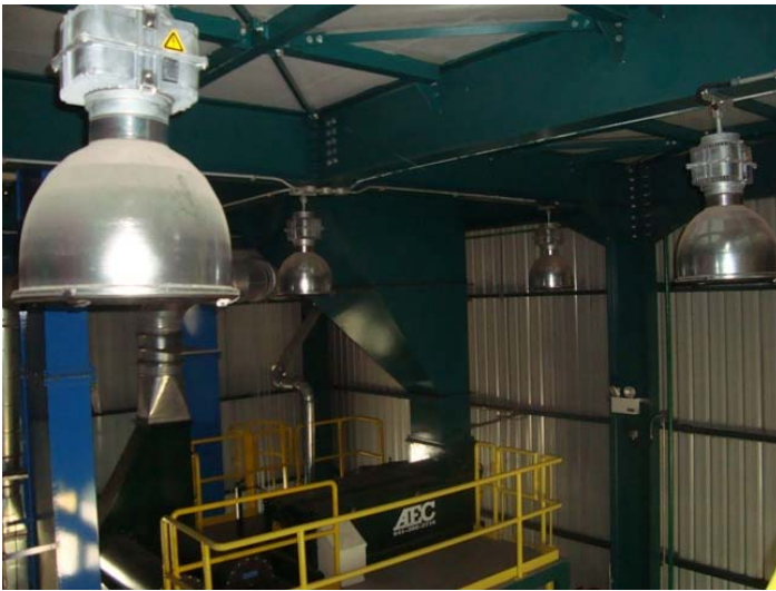
High bay Industrial Lighting installation
