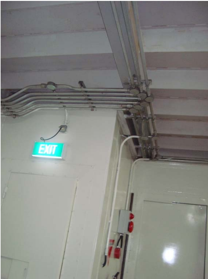
Fire Alarm System, EXIT lamp installation and electrical piping
